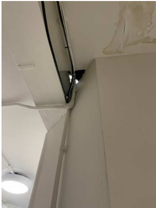
6 lift containment not sealed
