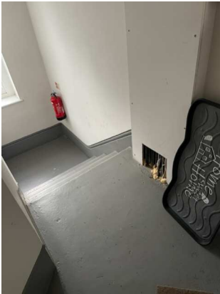
5 open services duct on internal fire landing
