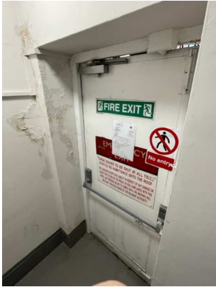
10 escape door between stairs to flat roof does not seal
