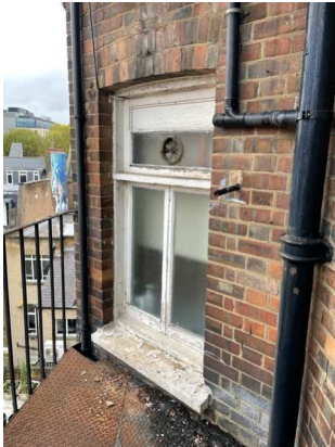
3 non-fire rated window on external escape landing
