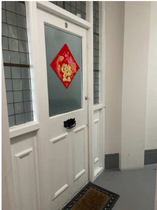
7 non fire-rated flat front door and side lights
