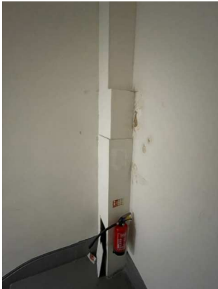
4 open services duct on internal fire landing
