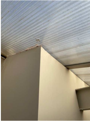
11 lift compartment not sealed at roof level
