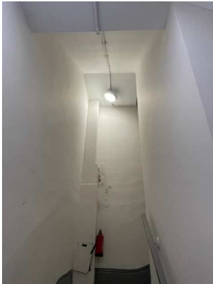
8 badly installed escape lighting
