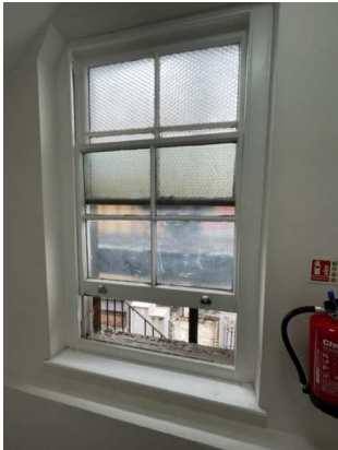
2 open window between stairs many panes not fire rated
